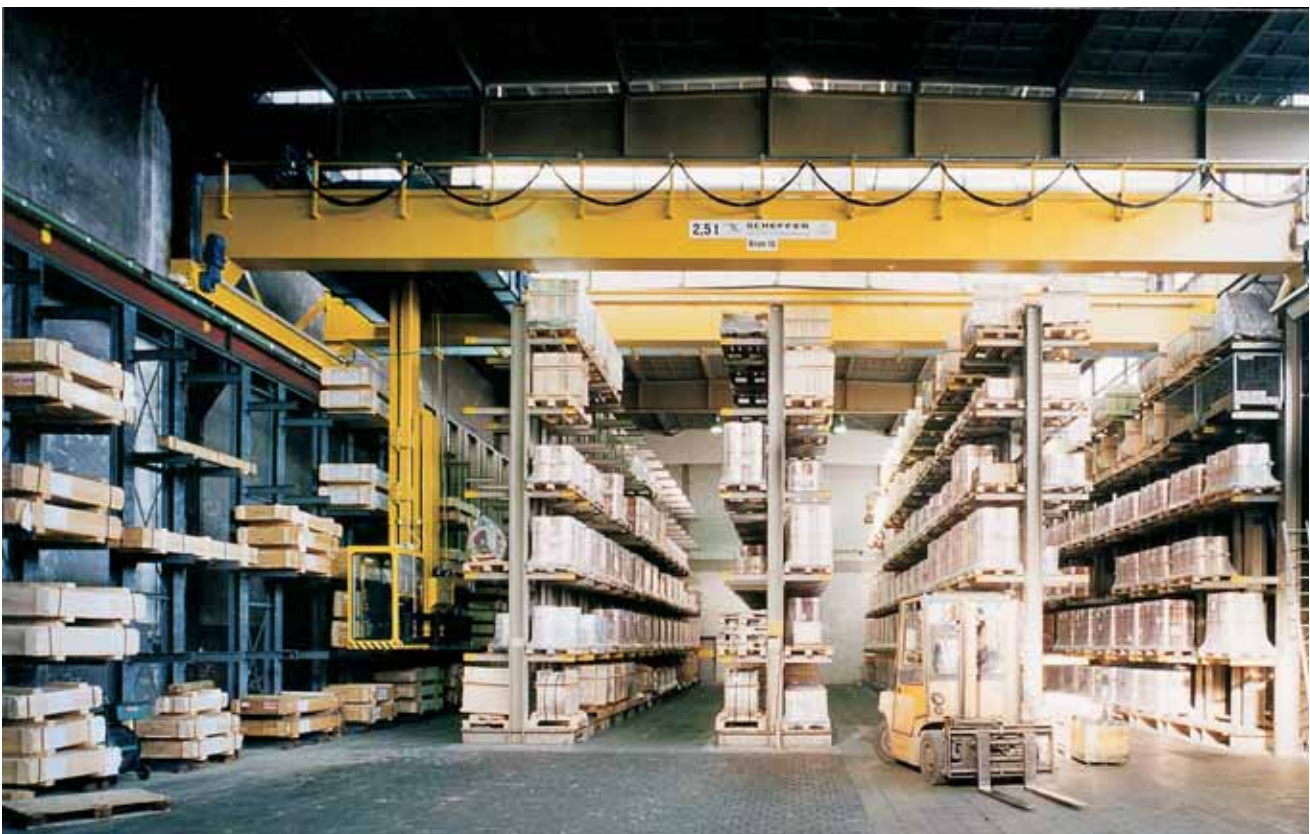
for stacker crane electrification.
